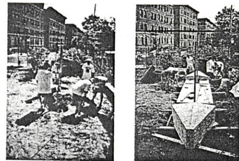
The "boat" under construction
